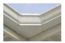
The extended front end of the **Extreme Miter™** Inside Gutter Corner provides an enlarged catch basin, directing water away from the front edge and
